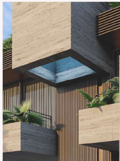
IROKO FACADE CLADDING
